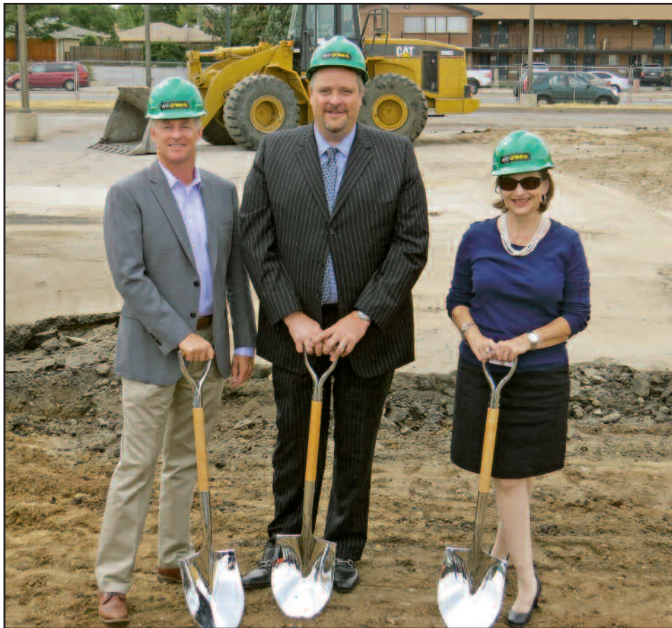
Groundbreaking: Formerly known as Murray BMW, Sonic Automotive's new BMW store is scheduled to open by this time next year on the site of a former Chevrolet dealership on Colorado Boulevard. The existing buildings on this site are in the process of being demolished and the new BMW dealership will be erected in their place. From left to right: Todd Guthrie, President of W.E. O'Neill Construction Company of Colorado; Bryan Haarhues, General Manager Sonic Automotive's BMW Store; and Valerie Kerns, aide to Denver Councilman Paul Kashmann. For more information, visit murraybmwofdenver.com .
